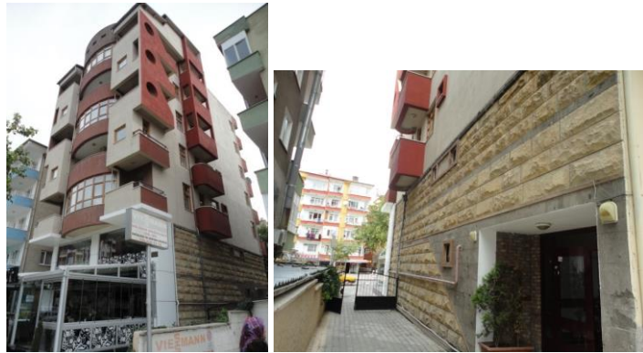
Picture 37. Ozlem apartment Store Facade and Details of the entrance
