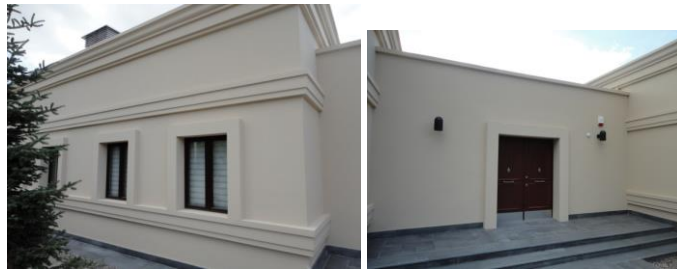
Picture 22. Facade details of the guesthouse
