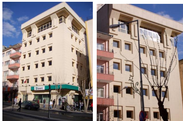
Picture 15. Ayhan Sahenk Boulevard facade of Garanti Bankasi Nigde Branch and details of the facade elements
